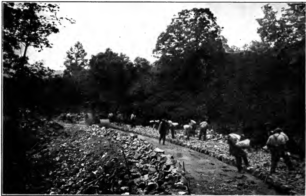
LAYING THE TELFERD BASE OF A BITUMINOUS MACADAM PAVEMENT IN A HEAVILY TRAVELED SECTION OF THE INTERSTATE PALISADES PARK RESERVATION, NEW JERSEY
